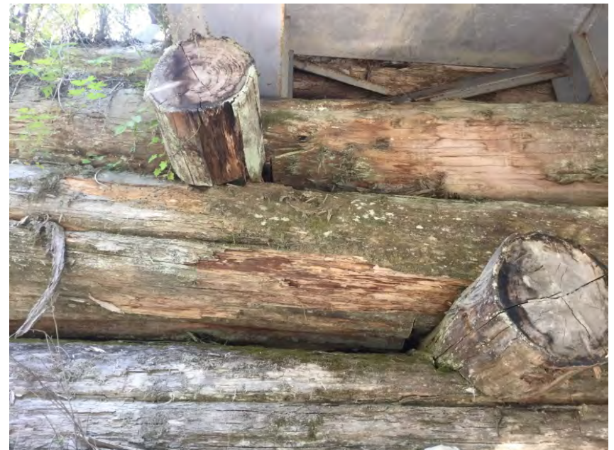
Log crib condition
