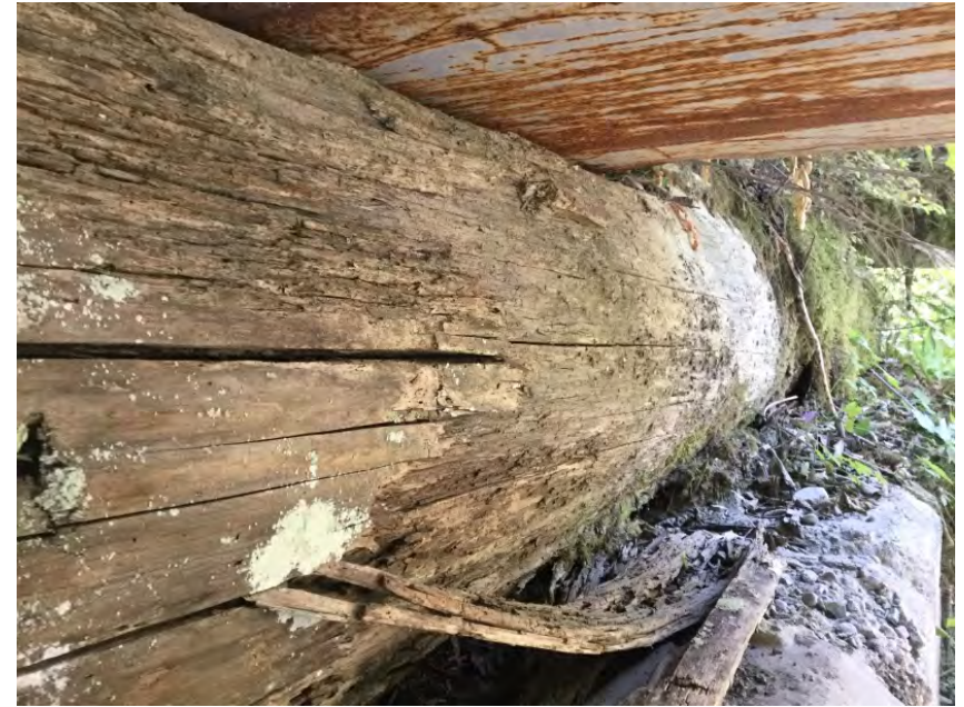
Right bank log sill condition
