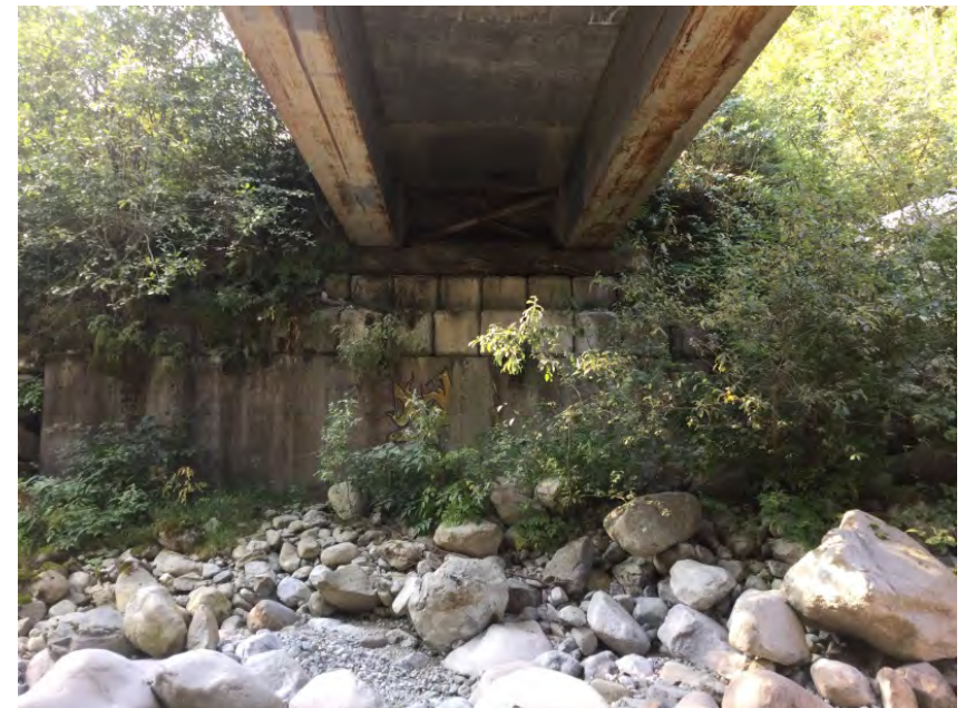
Right Bank Abutment when facing downstream
